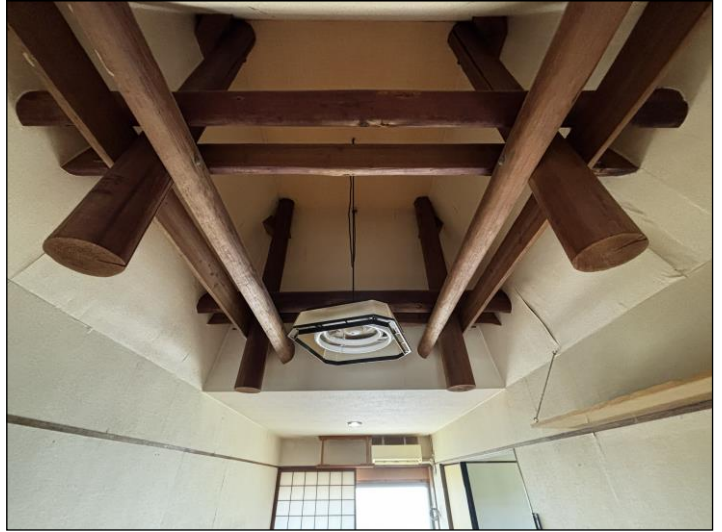
洋室①天井
